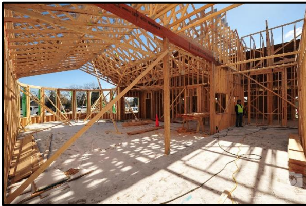
Figure 7 & 8 – Roof Trusses and Shear Walls, Panel Installation
